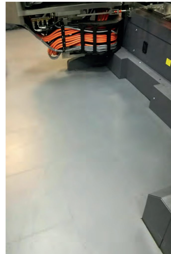
Textured tile 7mm & 9mm Dovetail interlock
