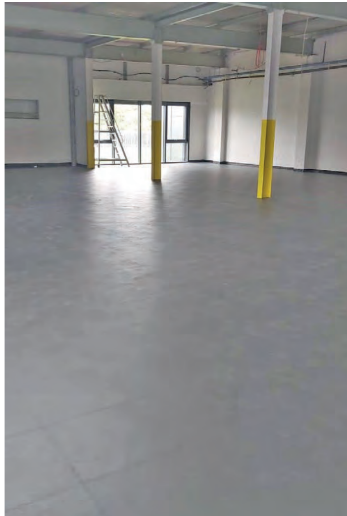
Textured tile 7mm & 9mm Dovetail interlock
