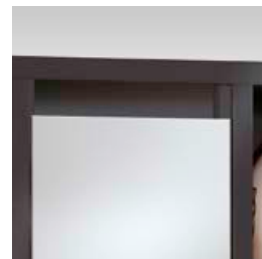
Doors shortened at the top for slot
